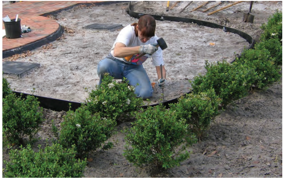
Installation of Super-Edg with stakes prior to planting.
